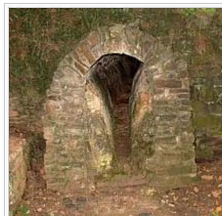
A portion of the ancient Roman **Eifel aqueduct** in Germany. In service for about 180 years, a deposit of scale up to 20cm thick built up within it.
