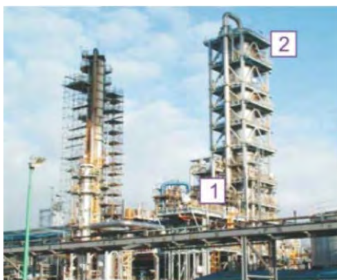
Acetic acid production facility (1: reactor, 2: distillation column) Photo provided BP Chemicals Inc.
